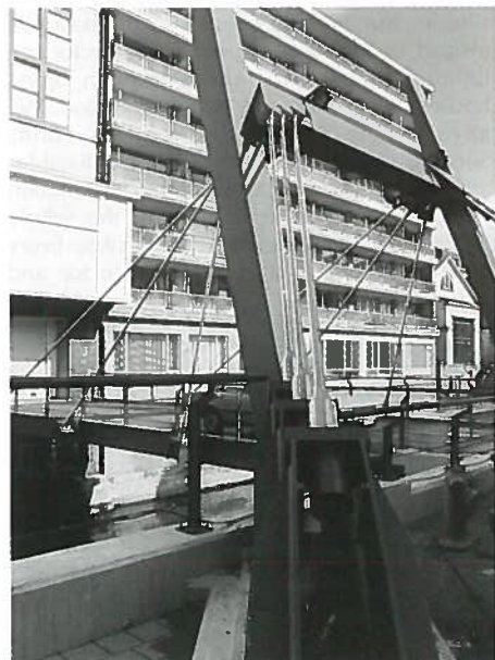
A new bridge provides access for scenery.
